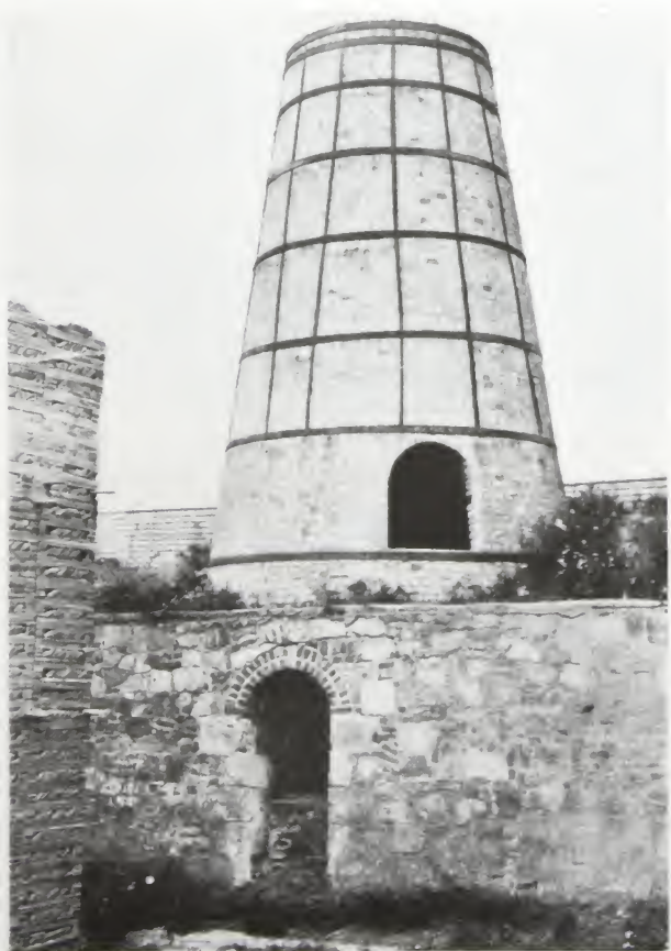
One of the early cement kilns erected in England by William Aspdin about 1850.
